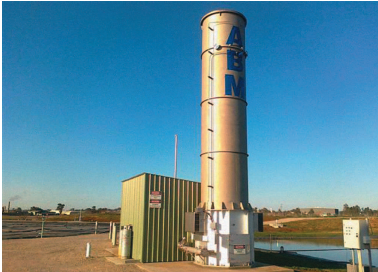
Enclosed Biogas Flare for combustion of methane produced from anaerobic waste water treatment ©Teys Australia (Wagga Wagga)
