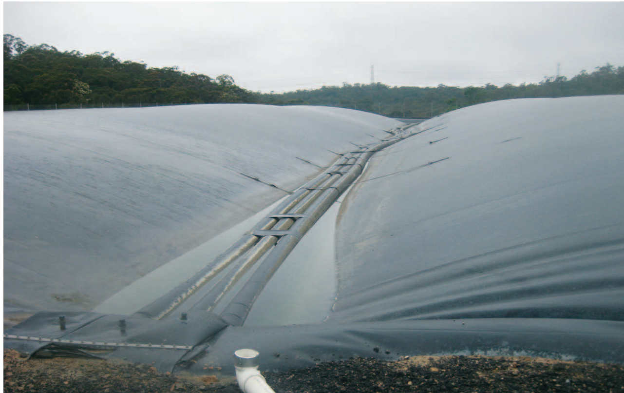
Stormwater removal system off CAL cover ©MINTRAC courtesy of Camilleri Stockfeed Pty Ltd
