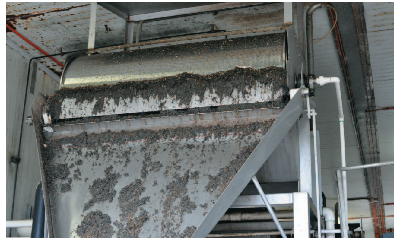
Effluent exiting over DAF weir ©MINTRAC courtesy of Big River Pork
