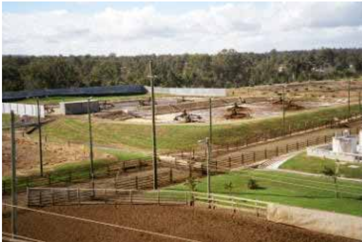
Aerial aspect of a Wastewater Treatment Plant
