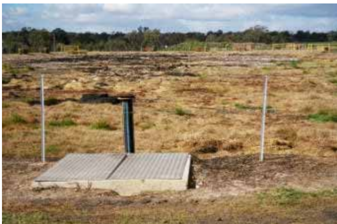
Anaerobic pond with a naturally formed crust
