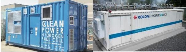
Figure 37: Containerised 200 kW and 1 MW Fuel Cell Modules with Pressurised H<sub>2</sub> Storage<sup>44</sup>
