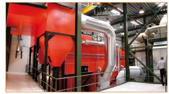
need for human involvement to generate thermal energy once the fuel has been delivered into the storage area. The boiler will command the fuel be fed to it depending on the demands that are, in turn, being placed on it from moment to moment.
