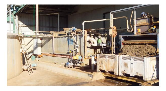
Photo 1: Typical dosed DAF and belt filter press for DAF float dewatering
