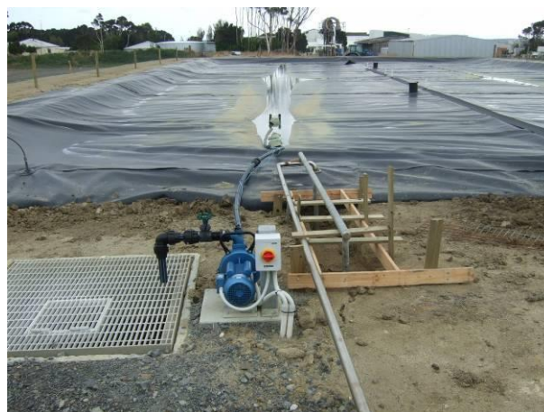
Photo 4: CAL showing stormwater removal
