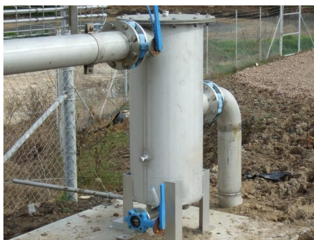
Image 14: Knockout pot in biogas train
