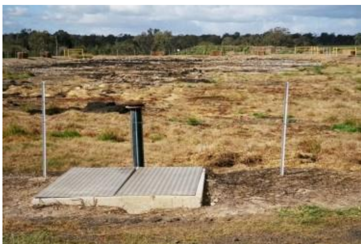
Image 1: A naturally crusted anaerobic pond processing wastewater from a large meat plant.
