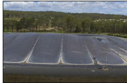
Covered Anaerobic Lagoon Image: Teys, Beenleigh
