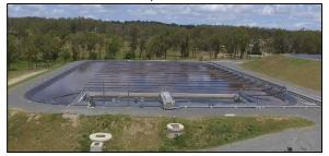
In **Continuous BNR processes**, nitrification and denitrification are performed in different parts of the reactor. An example is the Biolac process where although the denitrification zones are not separated by walls from the nitrification zones, there are distinct areas allocated for each reaction. This requires the constant circulation of flow between zones to complete the reaction. Image: Teys, Beenleigh
