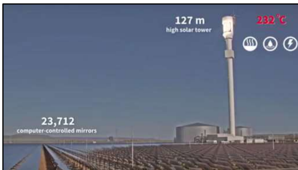
Figure 11: CST System generating up to 39 MWt for water desalination, greenhouse heating and power generation (1 MWe) at Sundrop Farms, South Australia 16, 17 .
