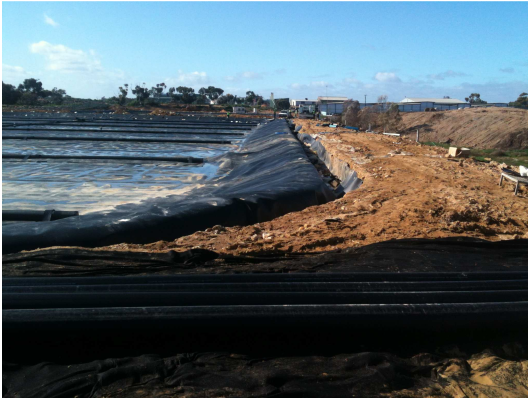
Figure 23: Anchor trench with cover installed in western CAL
