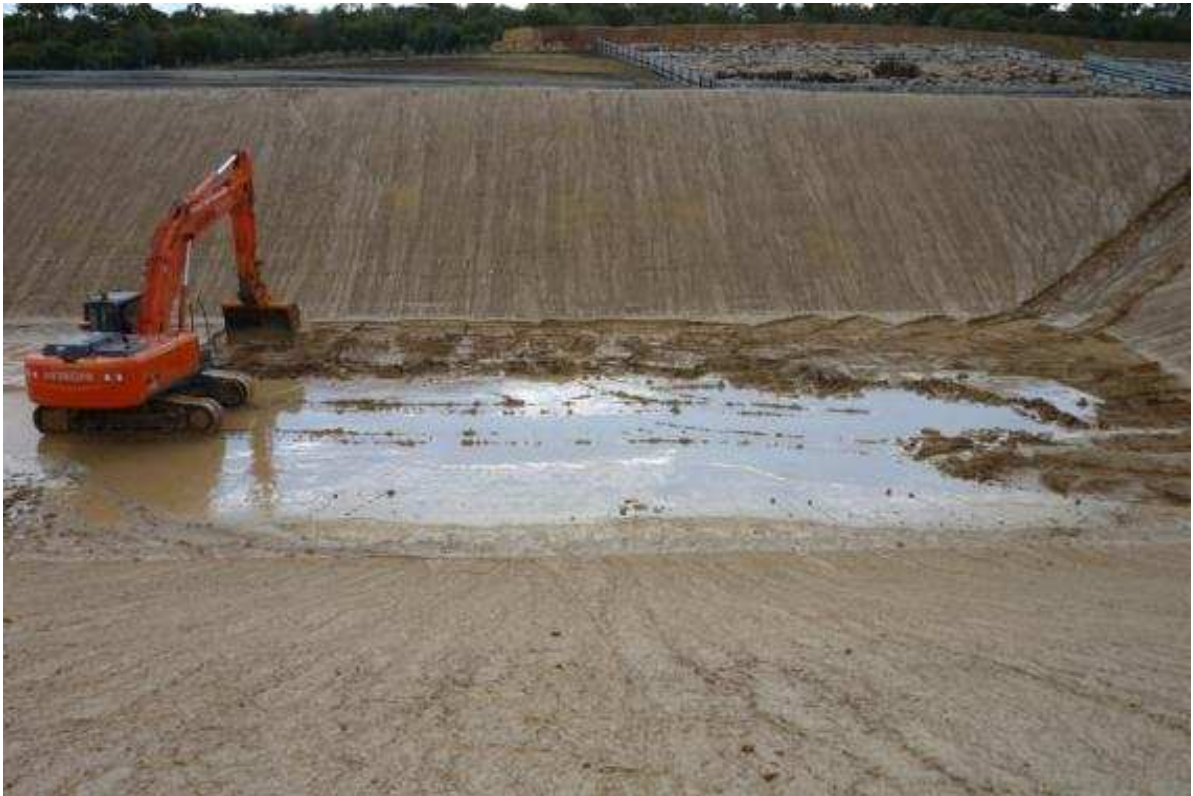
Figure 17: Re-working earthworks following rainfall
