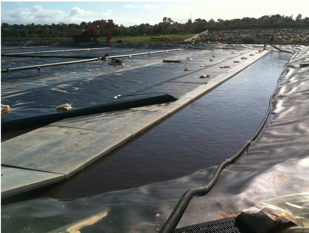
Figure 22: Installation of cover on western CAL using floating pontoon
