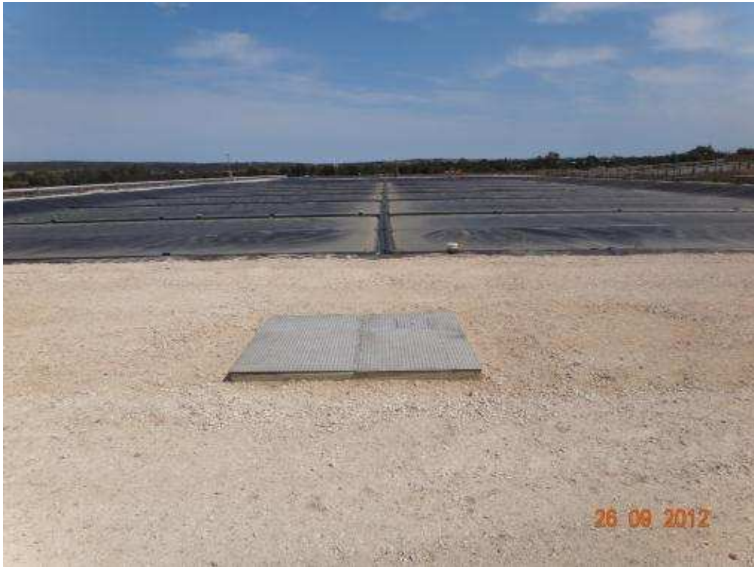
Figure 24: CAL cover (eastern CAL) prior to biogas generation
