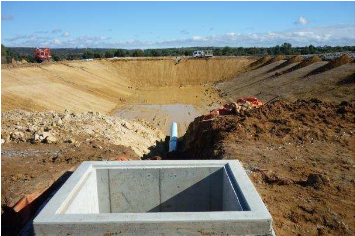
Figure 26: Eastern CAL outflow weir
