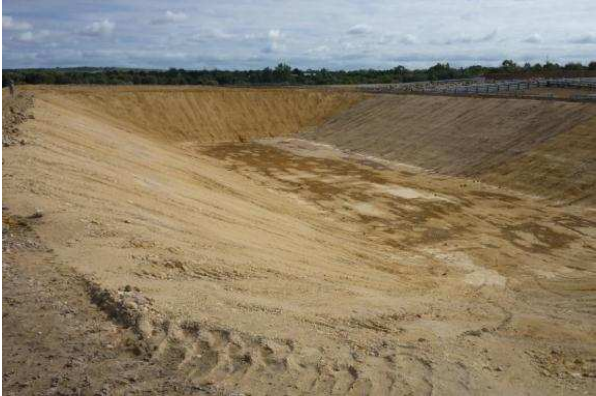
Figure 16: Bulk excavation of eastern CAL
