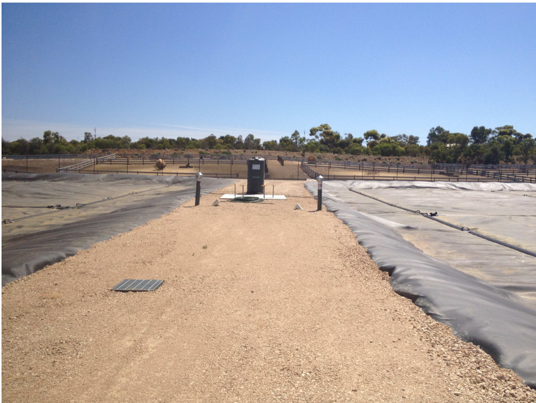
Figure 32: Central distribution weir and cover weight top-up water tank
