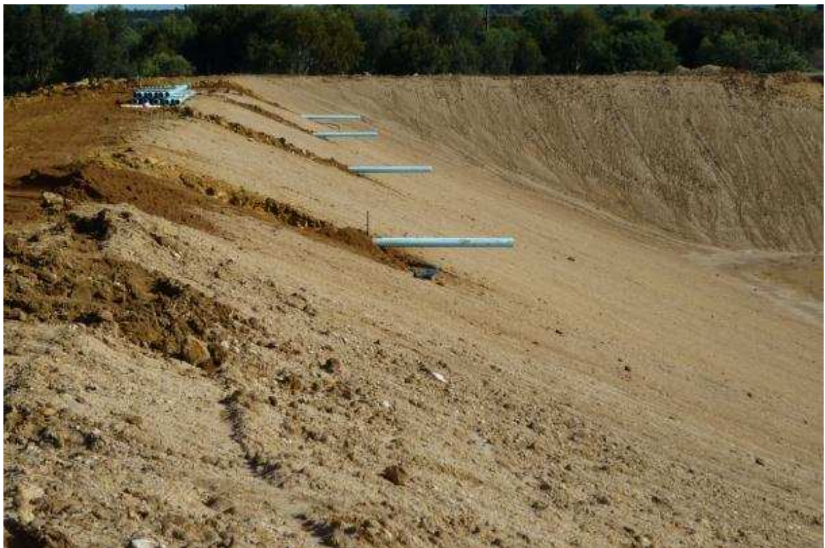
Figure 27: Sludge removal pipe penetrations on the western lagoon
