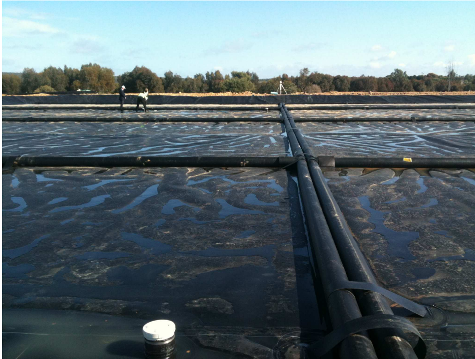
Figure 20: Cover weigh down system during construction
