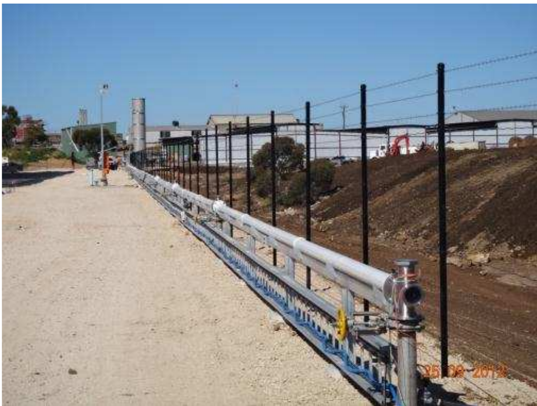
Figure 30: Pipe bridge located on outside of embankment
