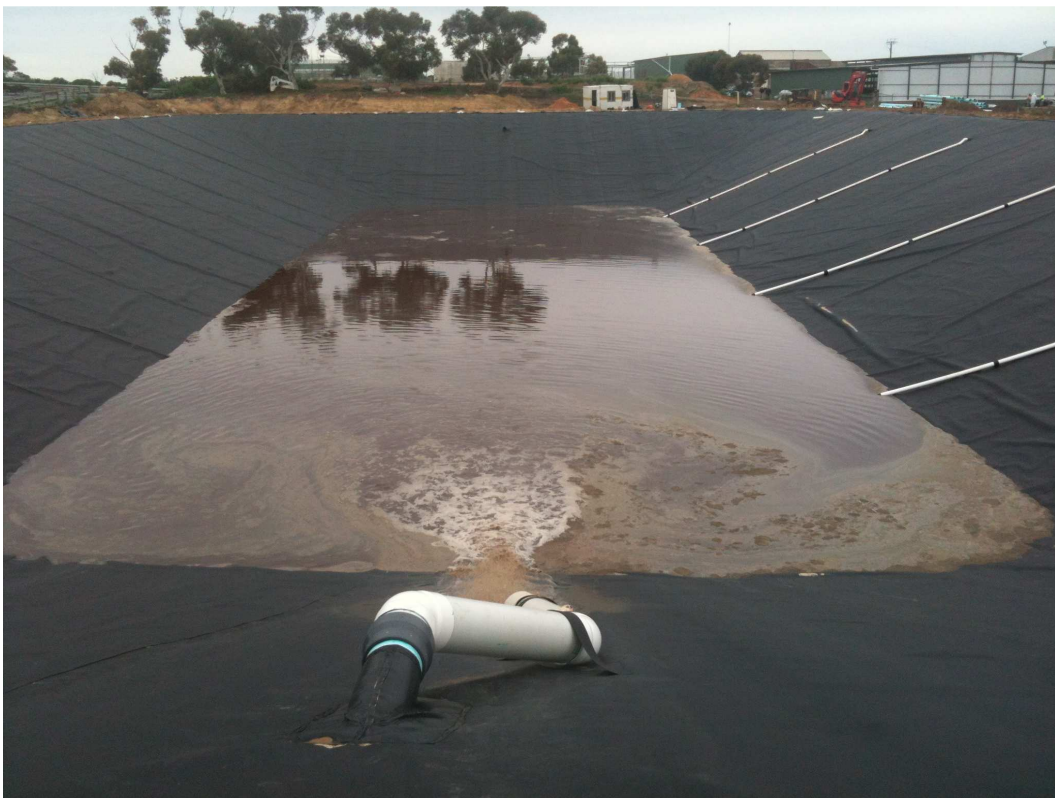
Figure 29: Inlet to eastern CAL during initial filling
