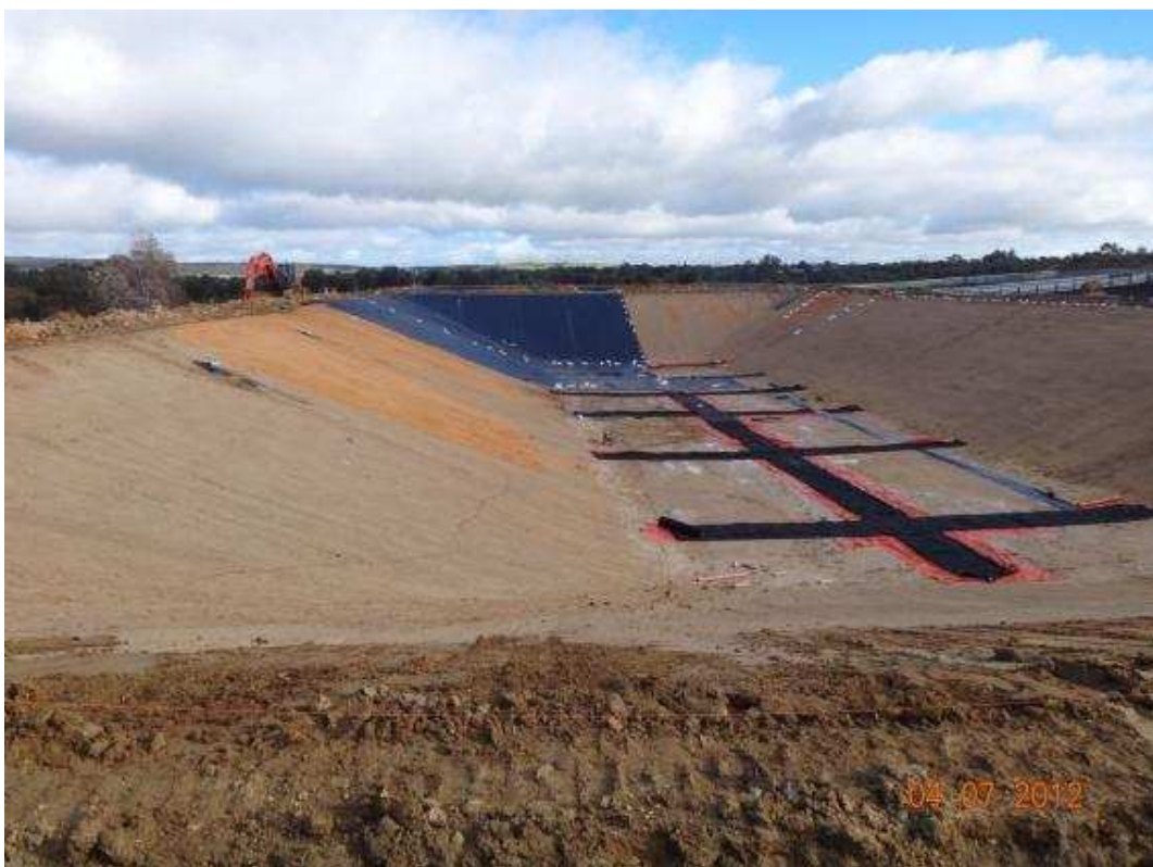
Figure 18: Leak detection system and commencement of lining (eastern pond)
