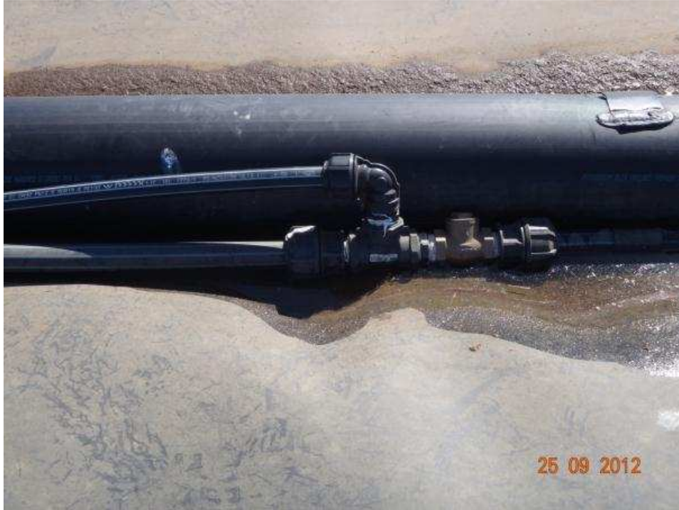
Figure 19: Rainwater removal system
