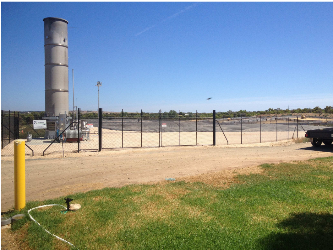
Figure 34: Flare and security fence
