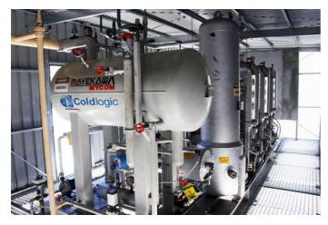
The basic concept of the AHP works on the basis that discharge gas from the high side of the ammonia refrigeration plant is drawn and recompressed by a high pressure compressor. This elevates the pressure and increases the temperature which in turn is passed through a heat exchanger where it transfers its heat to water on the other side.
