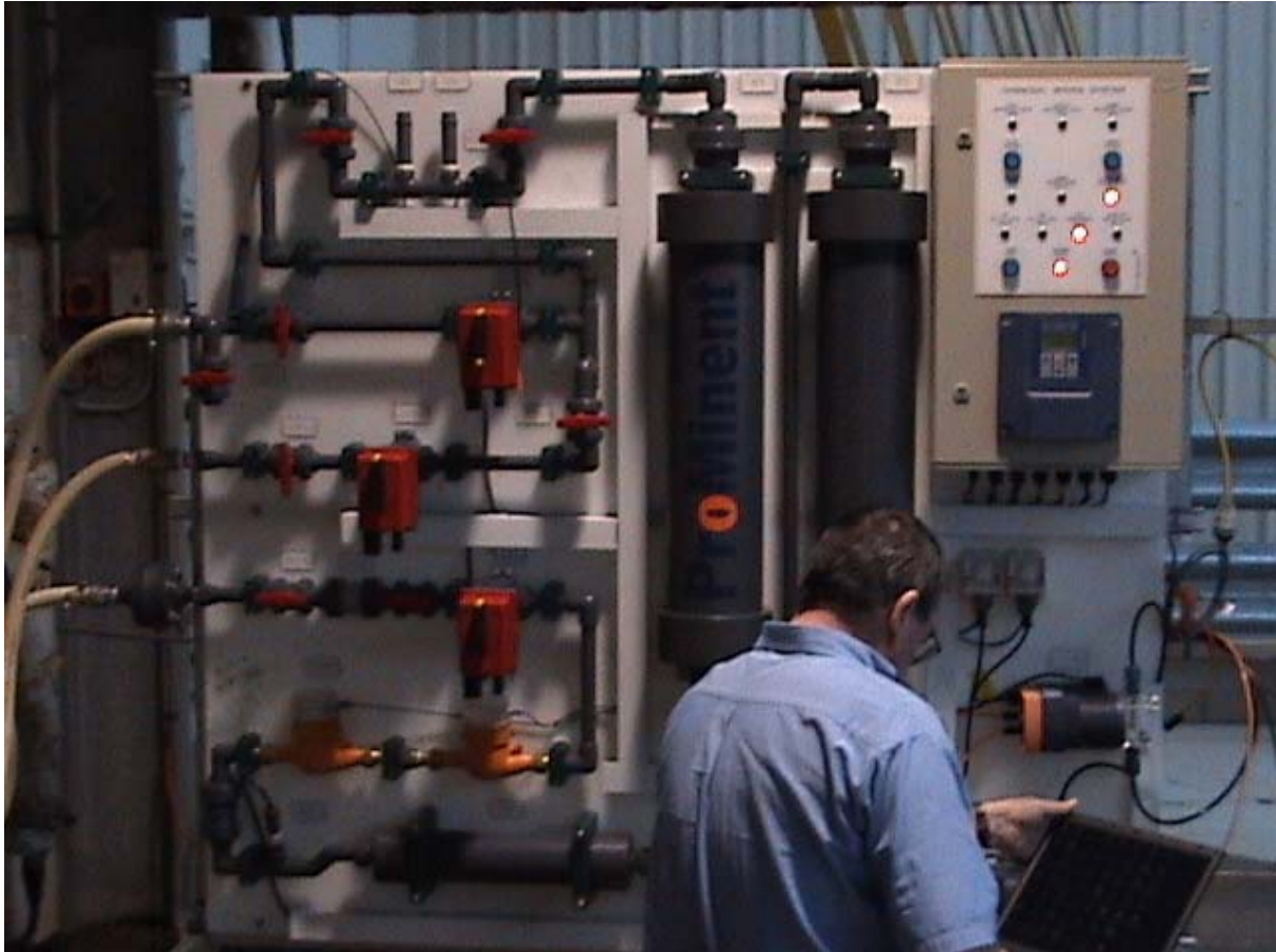
Figure 7 Installation of the Vibrex™ Dosing System by Grayson
