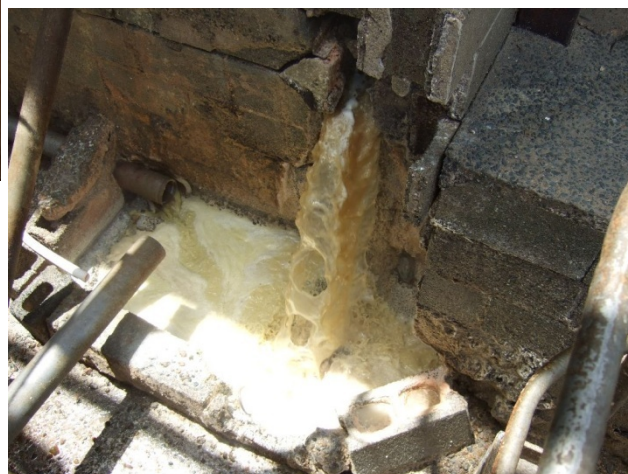
Photo 2. Stickwater drain with polisher stickwater entering at top left of drain and occasional tallow tank discharge at top centre. – also very strong waste streams.
