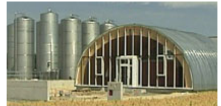
Figure 23 Biodiesel Plant in Austria
