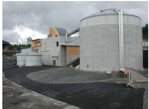
Figure 14 Exterior of the finished plant
