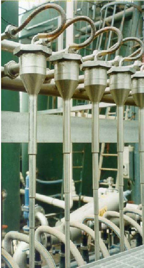
Figure 5 Meat Processing Plant No.1 – De-oiling and De-sanding Hydrocyclones
