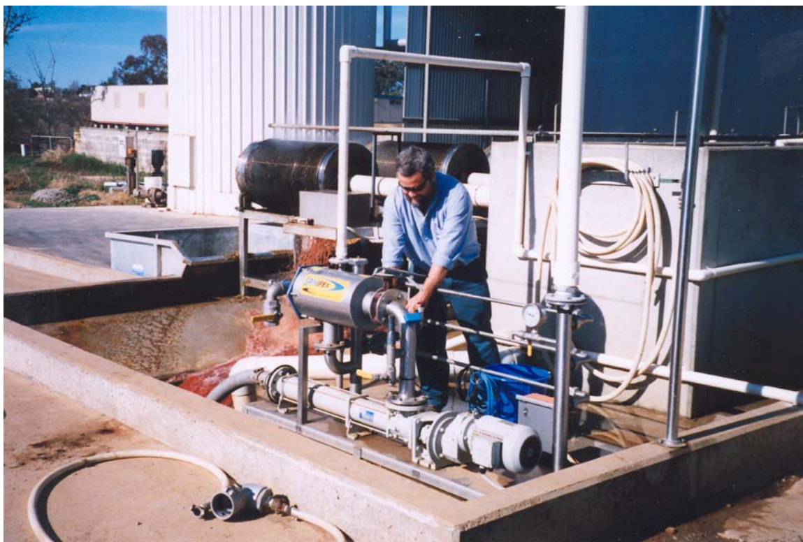
Figure 9 Sampling at Plant No.3 Hydrocyclone Installation
