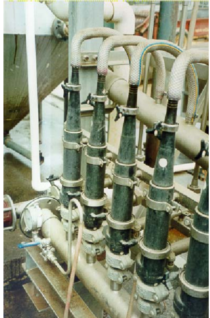
Figure 5 Meat Processing Plant No.1 – De-oiling and De-sanding Hydrocyclones
