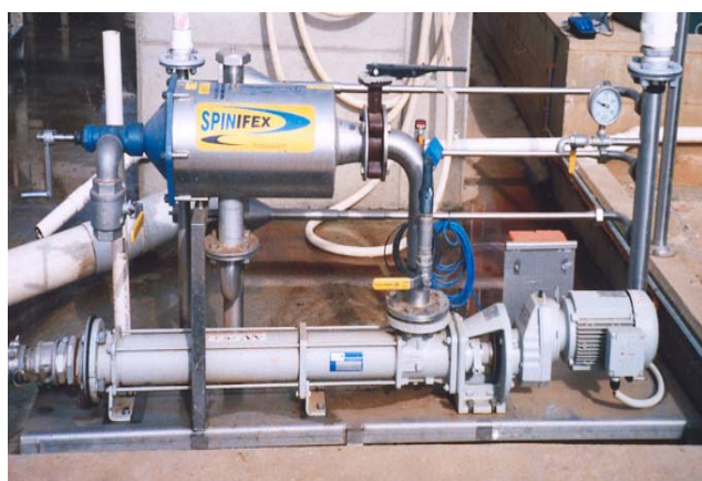
Figure 10 Meat Processing Plant No.3 – Hydrocyclone Installation
