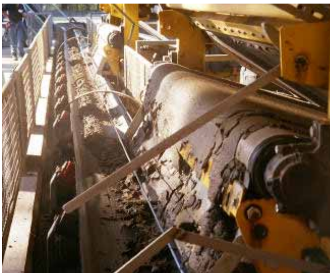
Belt press sludge
