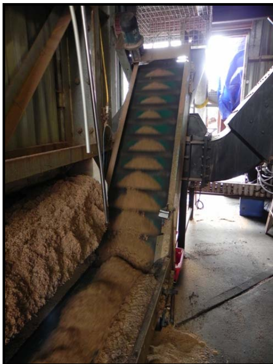
Sawdust feed conveyor system
