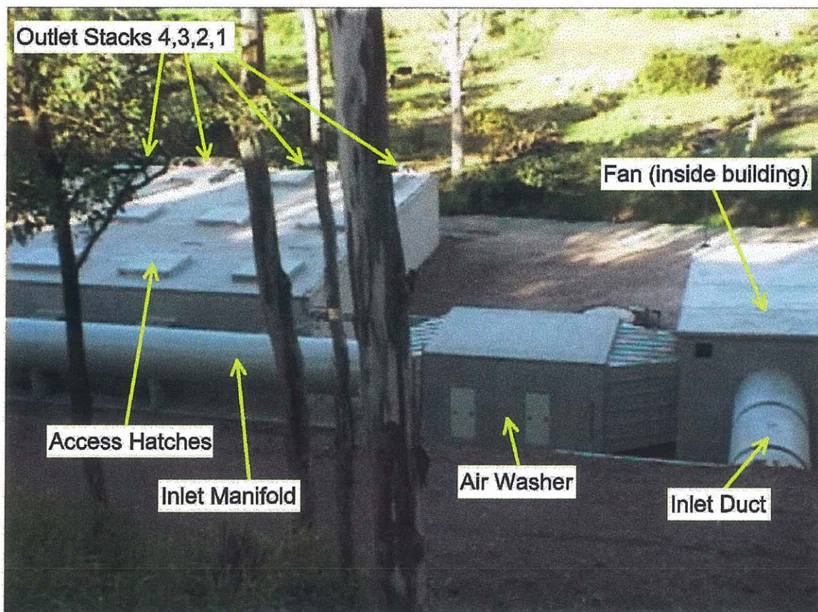
Figure 1 Major Components of the ACC Biofilter
