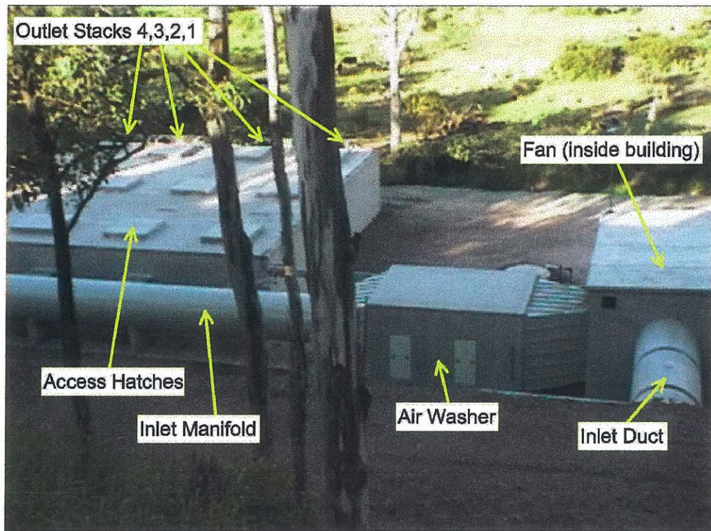
Figure 1 Major Components of the ACC Biofilter
