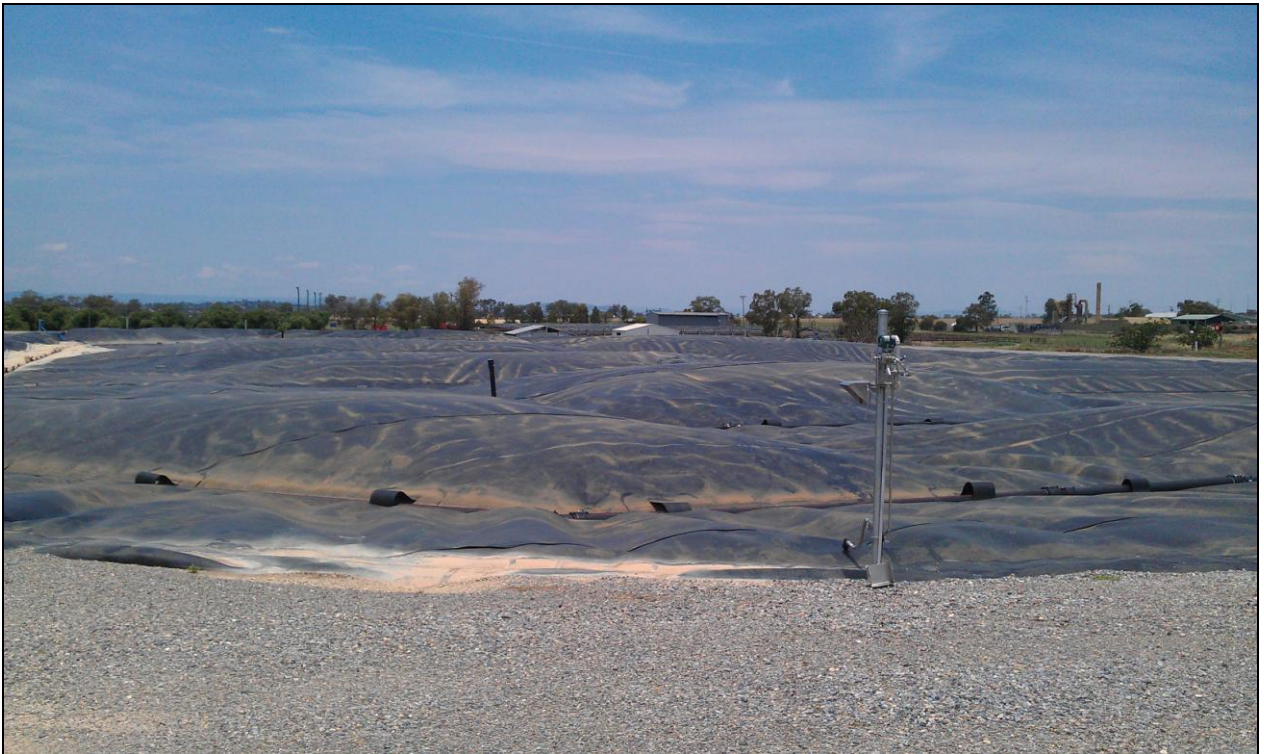
Photo 3.2 – CAL system at Abattoir A
