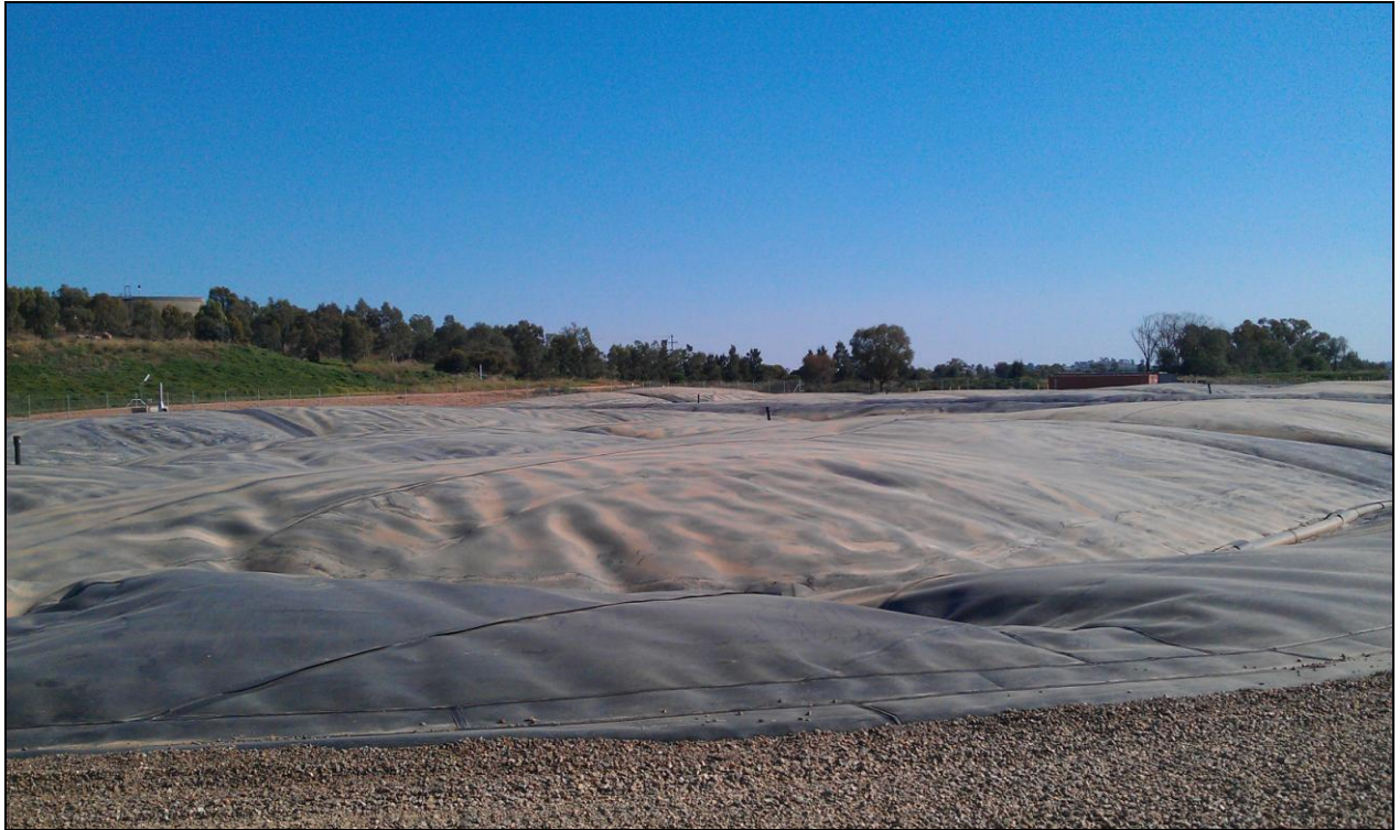
Photo 3.5 – CAL system at Abattoir B
