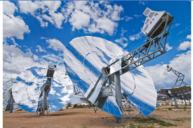
The Suncatcher, which uses a Stirling engine at the focal point of the parabolic mirror. It is an efficient way of generating electricity, although it can only work during the day 30
