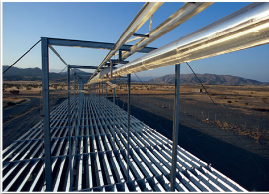
A Fresnel mirror. Solar energy is concentrated on the pipe running along the array (at top of picture) 29
