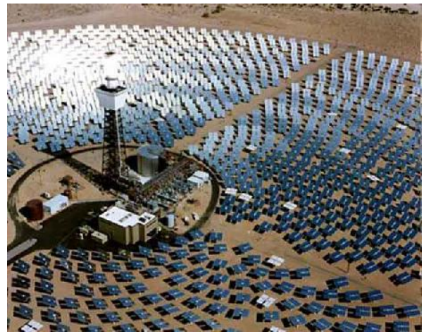
Solar tower, or heliostat, which uses an array of mirrors to concentrate solar energy on top of a tower 28
