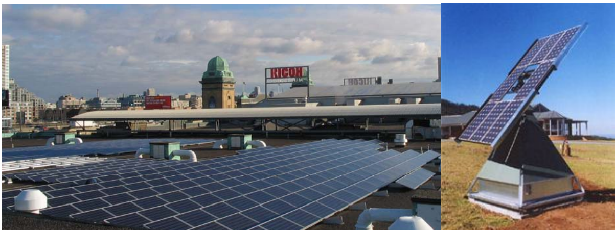
a) Fixed roof-top PV installation (Powersmart Solar); b) Ground mounted PV installation with dual-axis tracking (IT Power)
