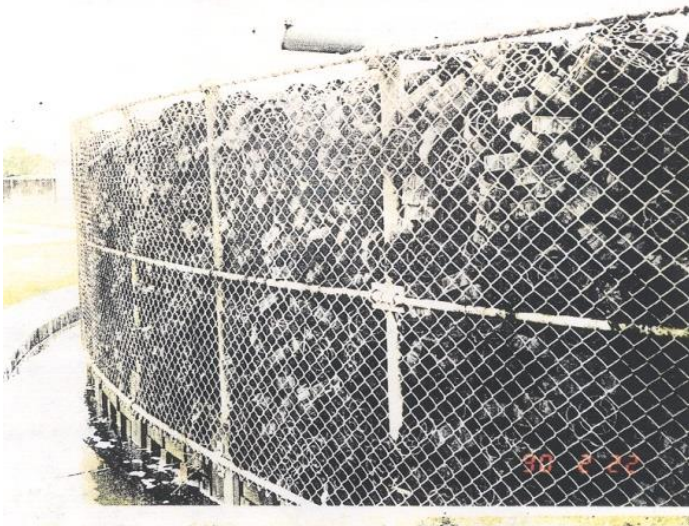
Figure 5: Mesh construction of modern plastic media TF
