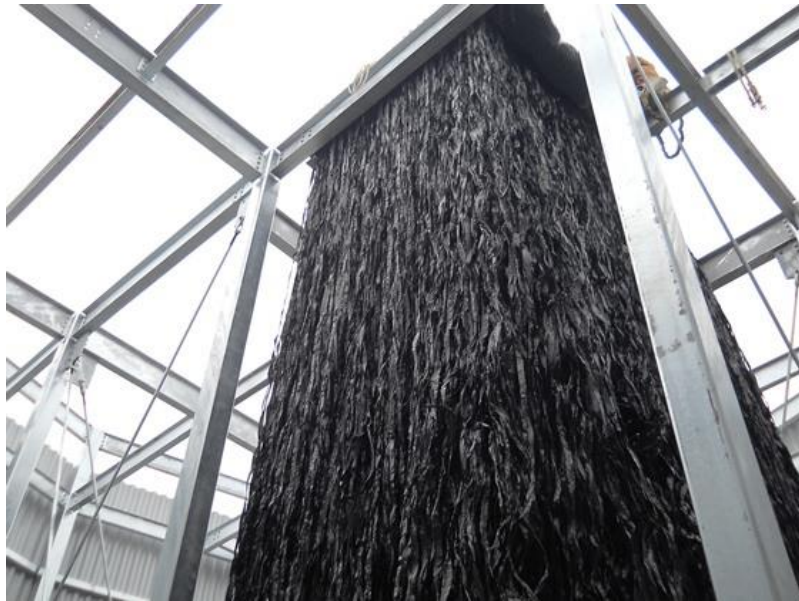
Figure 8: Raschig polypropylene strip media being installed, inside galvanized steel frame.
